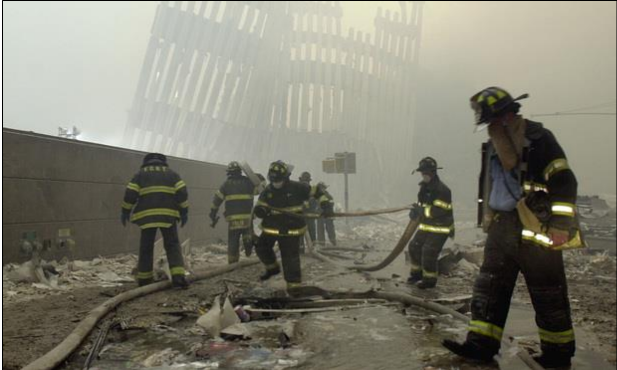
Firefighters work beneath the destroyed mullions, the vertical struts which once faced the soaring outer walls of the World Trade Center towers, after a terrorist attack on the twin towers in New York, on Sept. 11, 2001.
